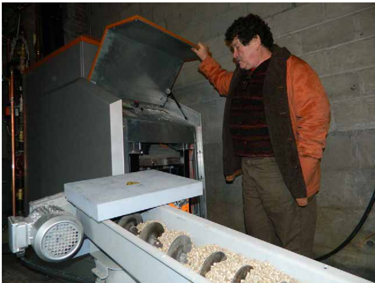
Greg Cox inspects the new Evoworld 100 biomass boiler installed at Vermont Farmers Food Center (Rutland, Vermont).
