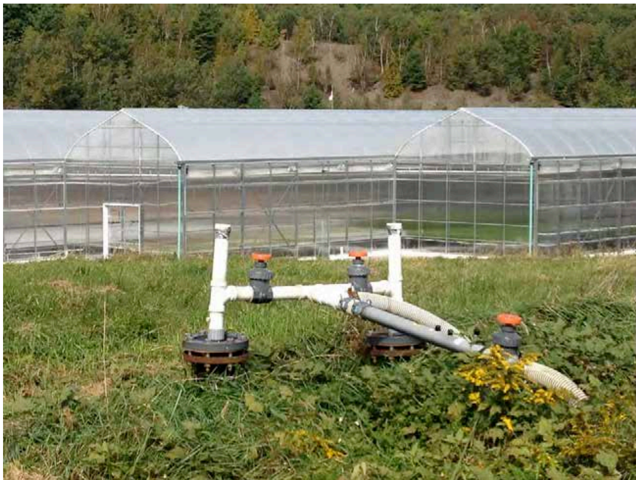
Landfill gas take-off plumbing is shown in the foreground with the CHE greenhouses in the background.
